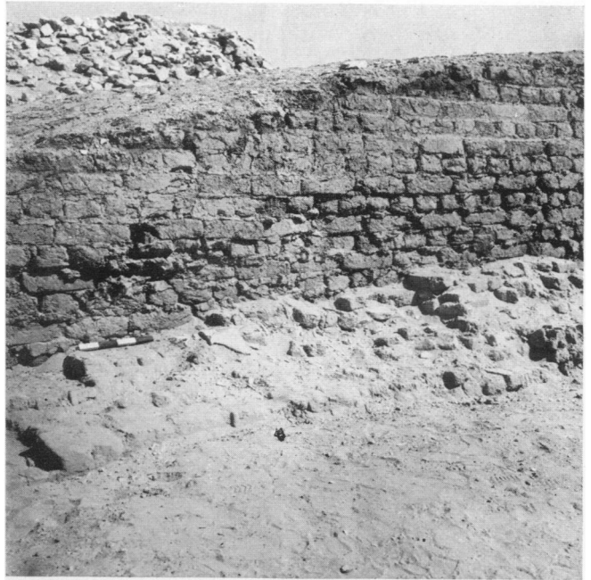
2. Inner wall of the ramp, from the south
